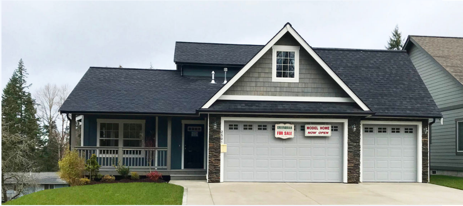
Pine Lodge with unfinished basement
